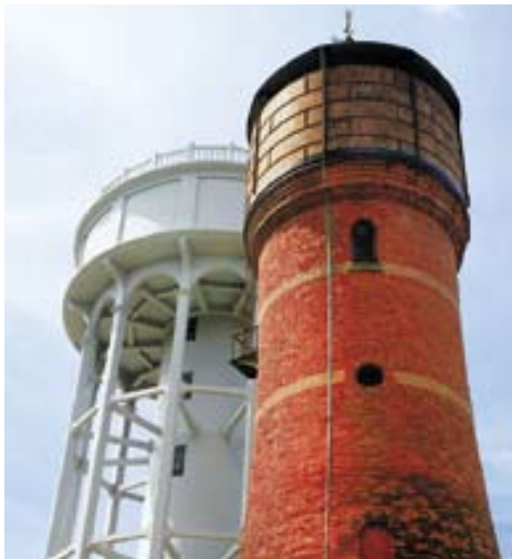
Rockwell Green Towers restoration, Wellington, UK.
